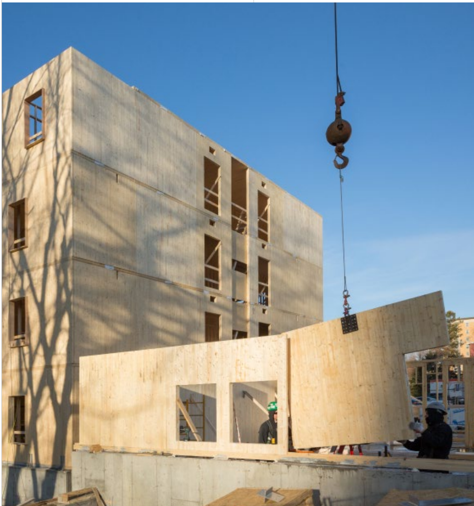
FIG 1: Open panel installation 70
