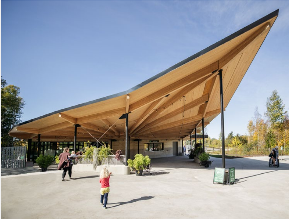
University of Alberta Botanic Garden Main Entry Pavilion, Edmonton, Alberta
