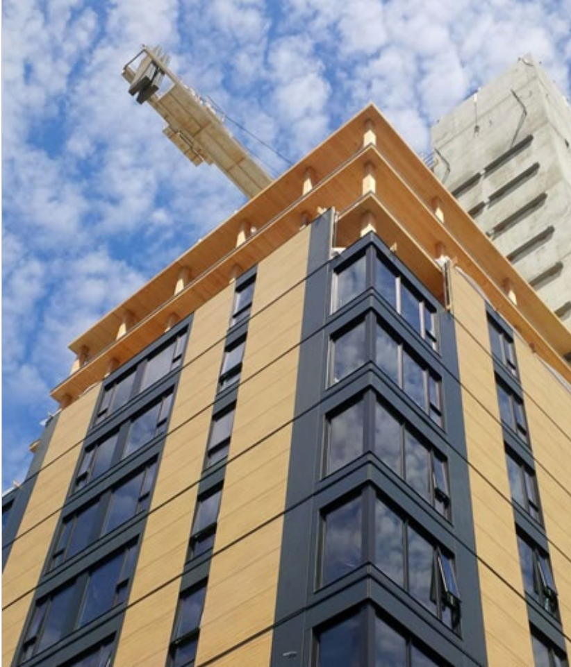
Brock Commons tall wood demonstration building Source: Natural Resources Canada
